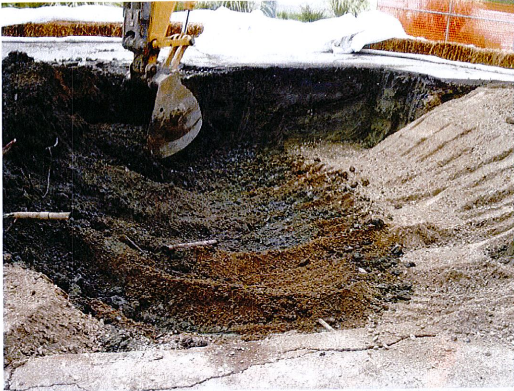
Backfilled western portion of excavation, removing impacted soil along southern wall
