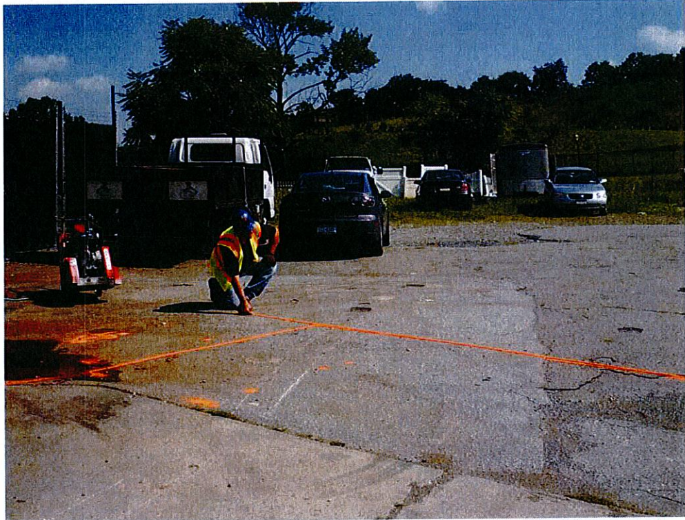
SAIC and ENTACT marking out excavation limits prior to breaking ground
