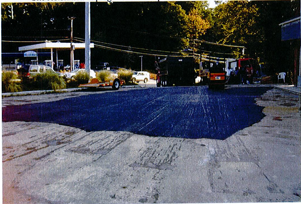
Site restoration complete
