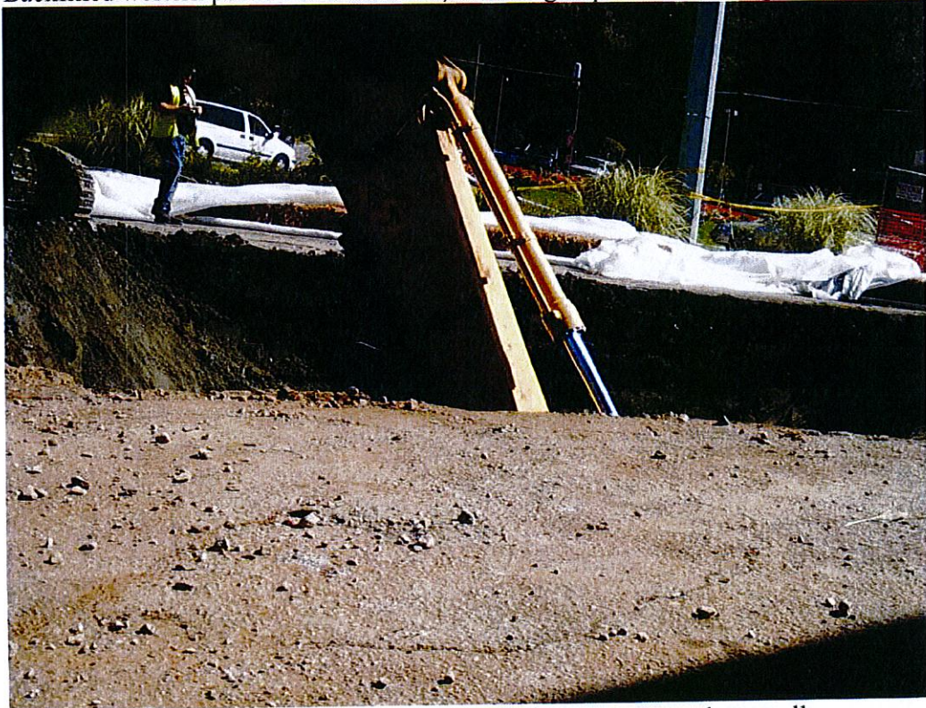
Excavator arm reaching a depth of 8 ft bgs along southern wall
