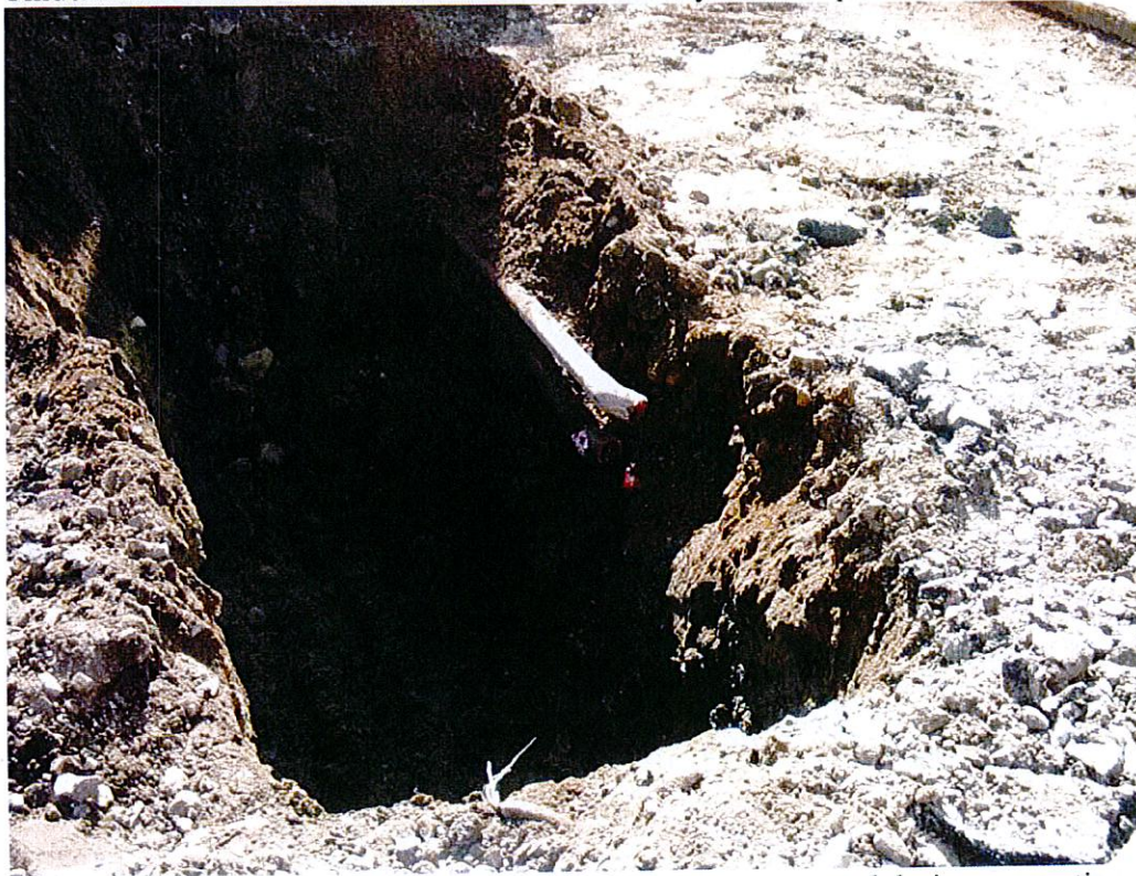
Old fiberglass product piping from dispenser area was removed during excavation
