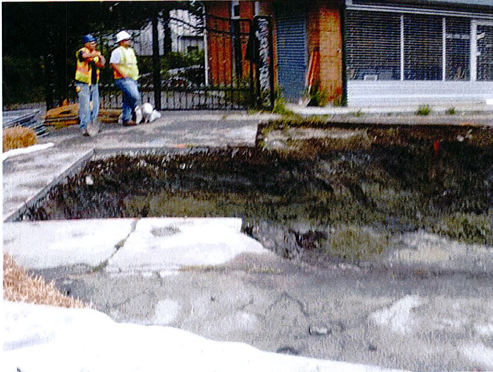
Proximity of excavation to station building
