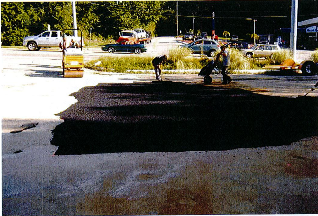
Site restoration in progress – new asphalt cover over excavation area
