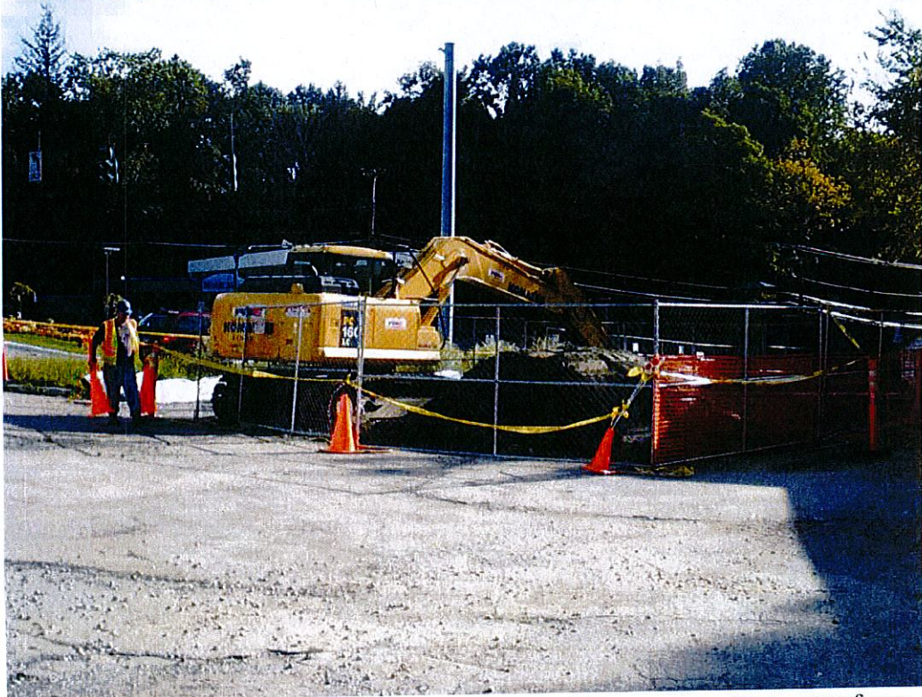
Excavation secured overnight by using temporary fencing, cones, tape, snow fence
