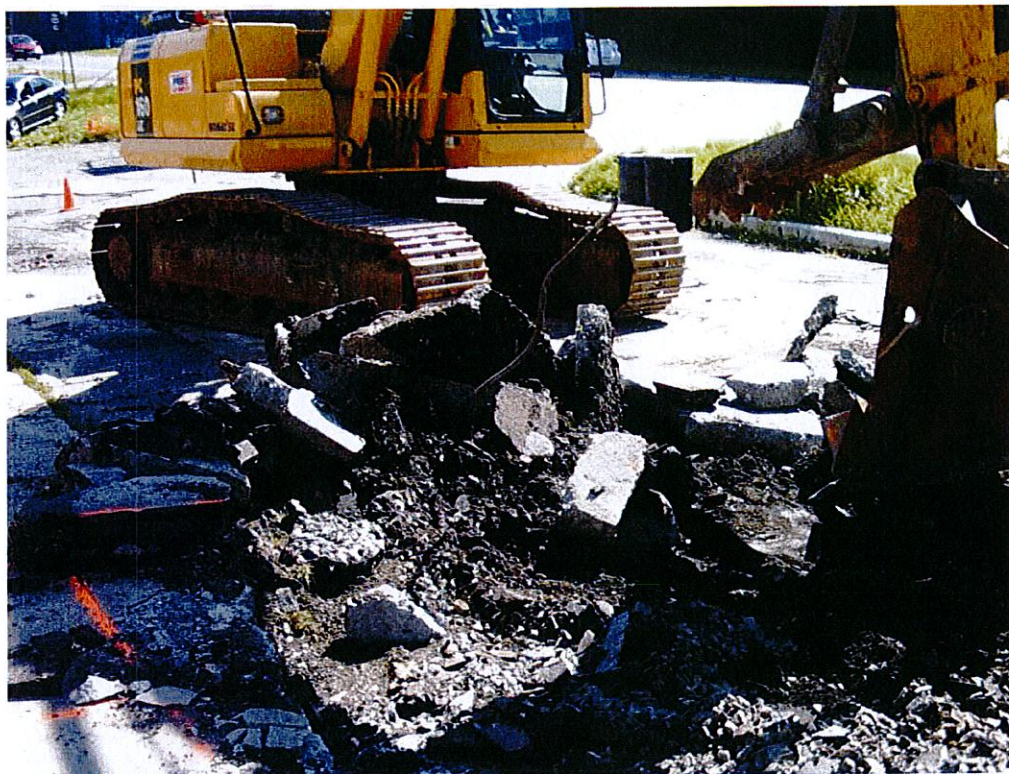
Unidentified utilities in excavation were evaluated by licensed plumber and electrician
