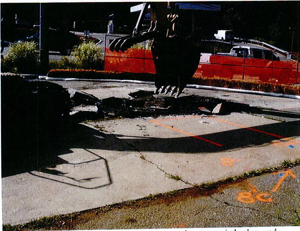
Excavator removing asphalt, erosion control measures in background
