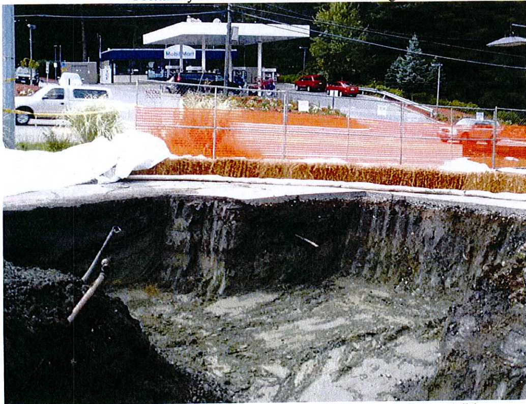
Final depth on western end of excavation – old dispenser piping visible
