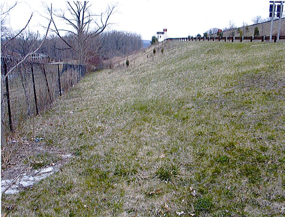
Photograph 41: Detail of embankment separating the Taconic State Parkway from the project site. View looking northwest.
