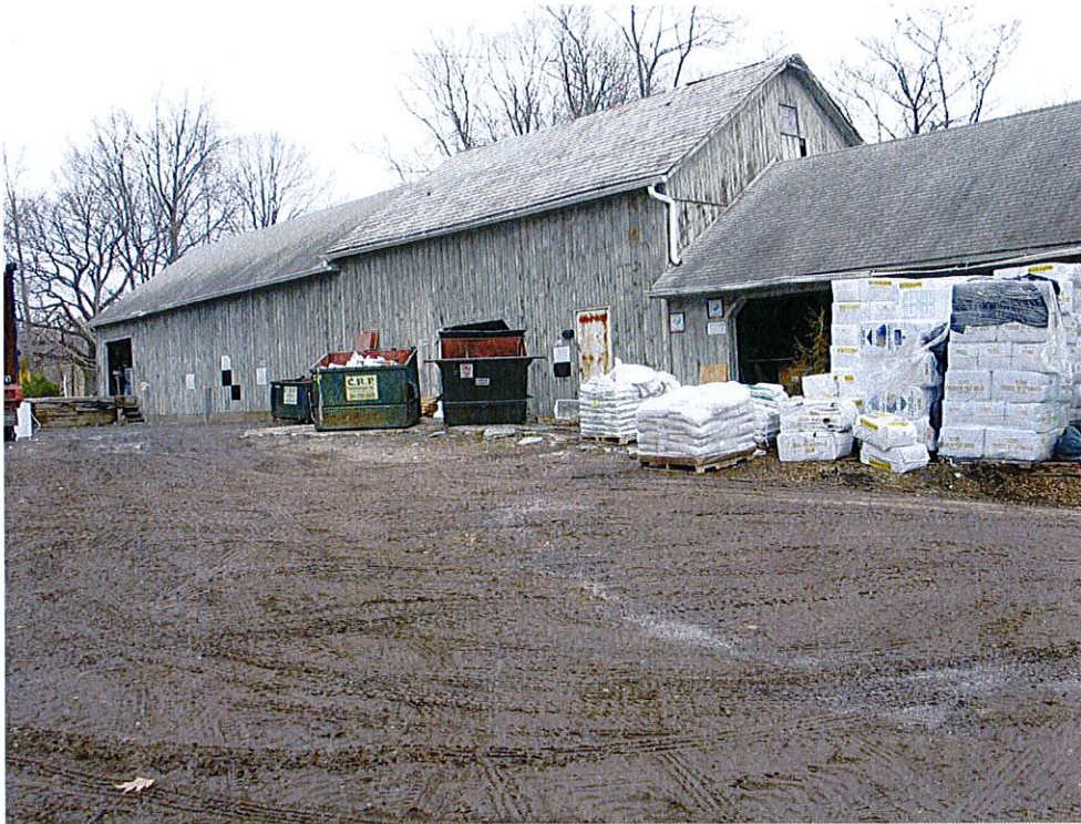
Photograph 15: Northwestern elevation of two story frame barn, comprised of three distinct sections. View looking northeast.
