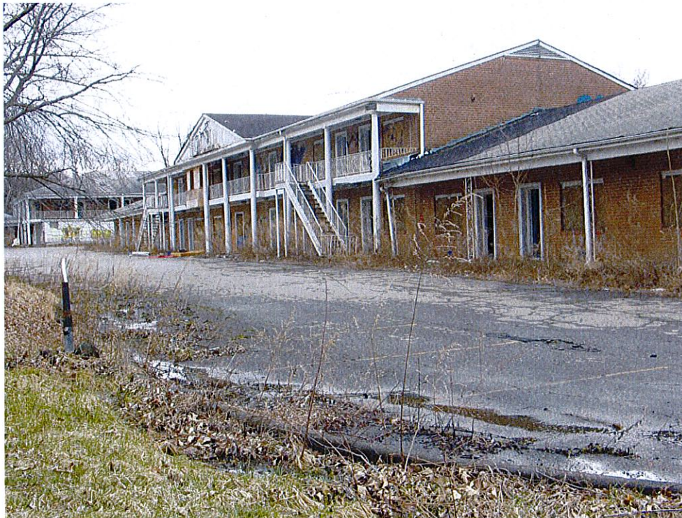
Photograph 18: Vacant motel complex showing eastern side of two former motel buildings. View looking southwest.
