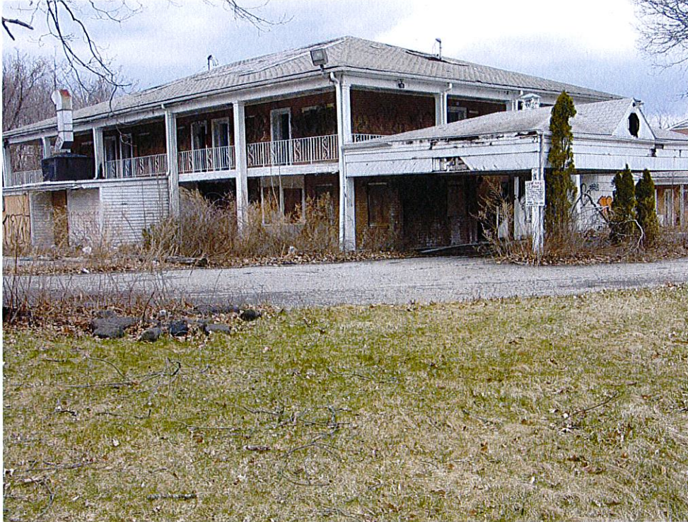
Photograph 19: Former two story office and restaurant building. View looking northwest.
