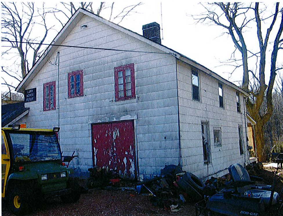
Photograph 8: Rear (north) elevation of former dwelling on Zino's Nursery and Landscaping and Anthony's Power Equipment property, now retrofitted and used to repair lawn mowers, showing wide double doors leading to workshop level. View looking southeast.
