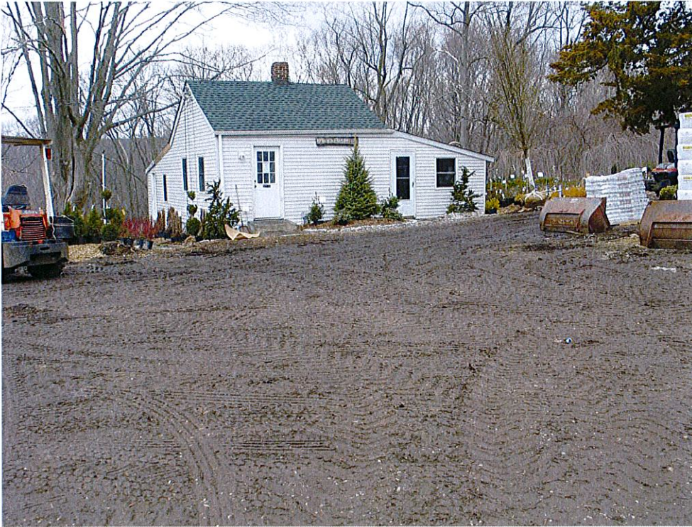
Photograph 13: Small, one story frame building used as an office for Zino's Nursery and Landscaping. View looking northwest.
