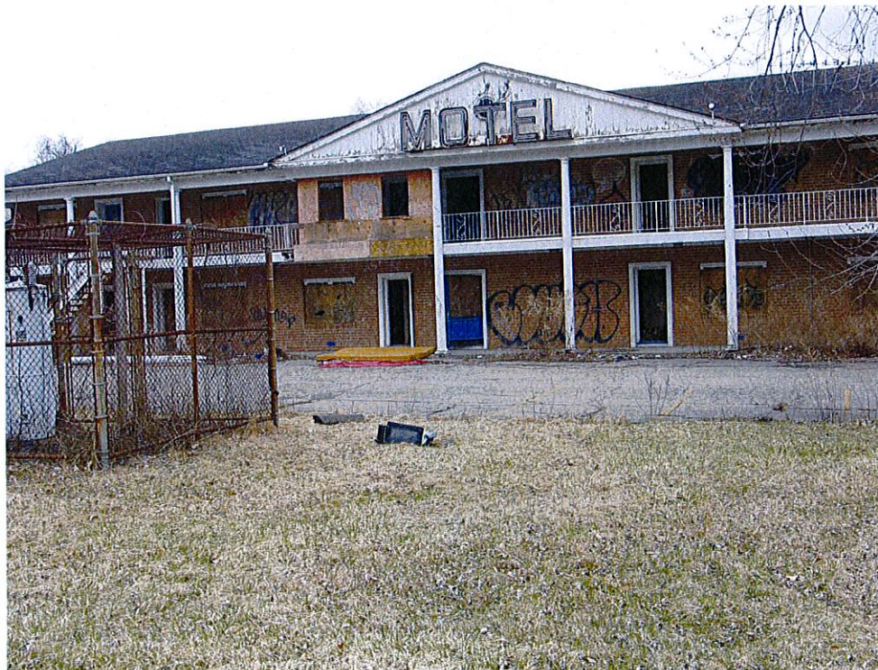
Photograph 20: Vacant motel showing eastern side of former motel building, where the rooms were located. View looking southwest.
