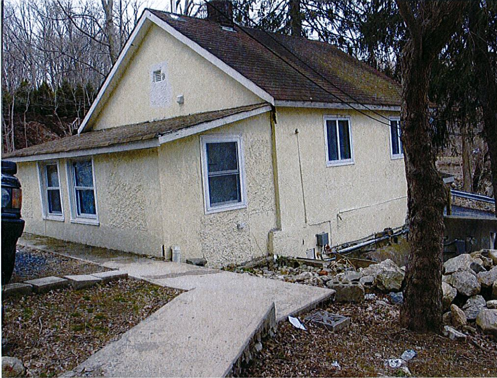
Photograph 3: Residence nearest Old Crompond Road showing one story addition off rear. View looking south.
