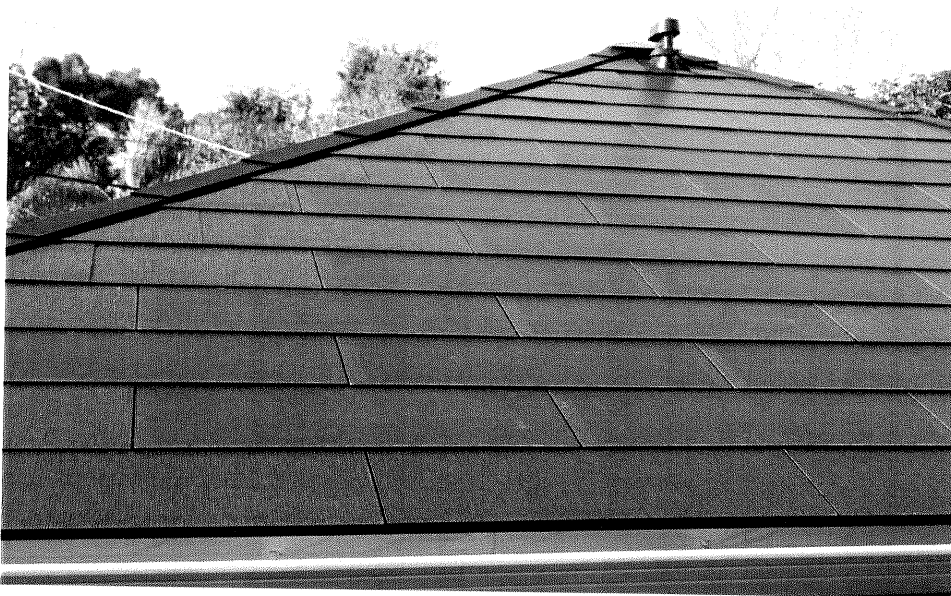
TYPICAL ROOF TEXTURE
