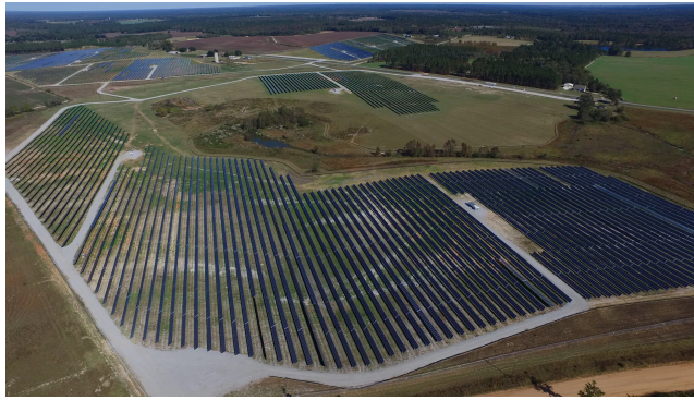
A solar farm developed by Hecate Energy in Millen, Ga. Many farms are built where abundant sunshine powers industrial-scale solar arrays and installations are farther away from sight lines. Hecate Energy
