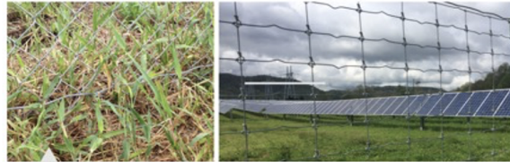
Comparison of a standard chain-link fence (left) with a wildlife-permeable fence (right). © Liz Kelley/TNC
