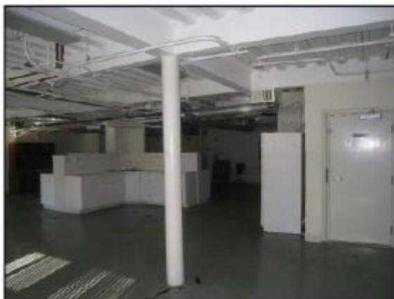
Open Basement Area
