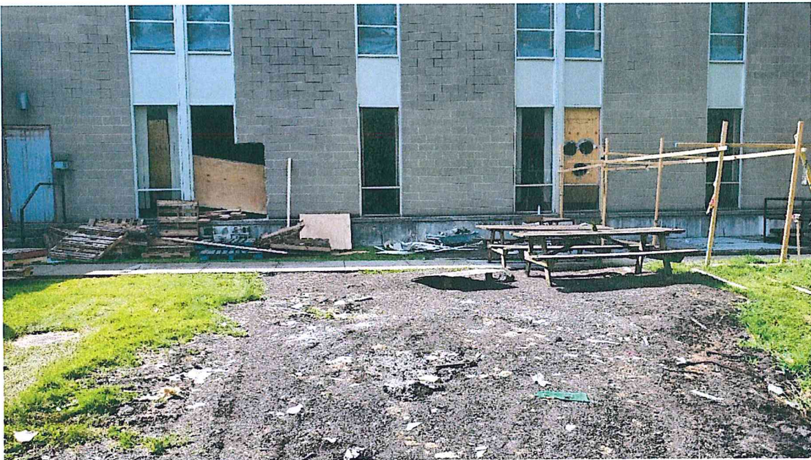
Photo 6 – Lower Level Demo
