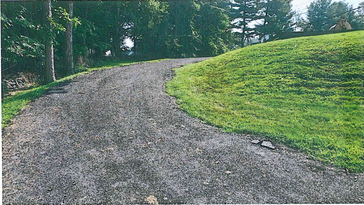
Photo 9 - Temporary Construction Access Road
