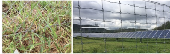
Comparison of a standard chain-link fence (left) with a wildlife-permeable fence (right). © Liz Kelley/TNC
