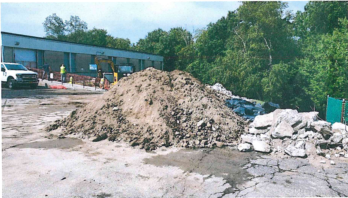
Photo 2 – Cut Material Stockpile – Clean Fill
