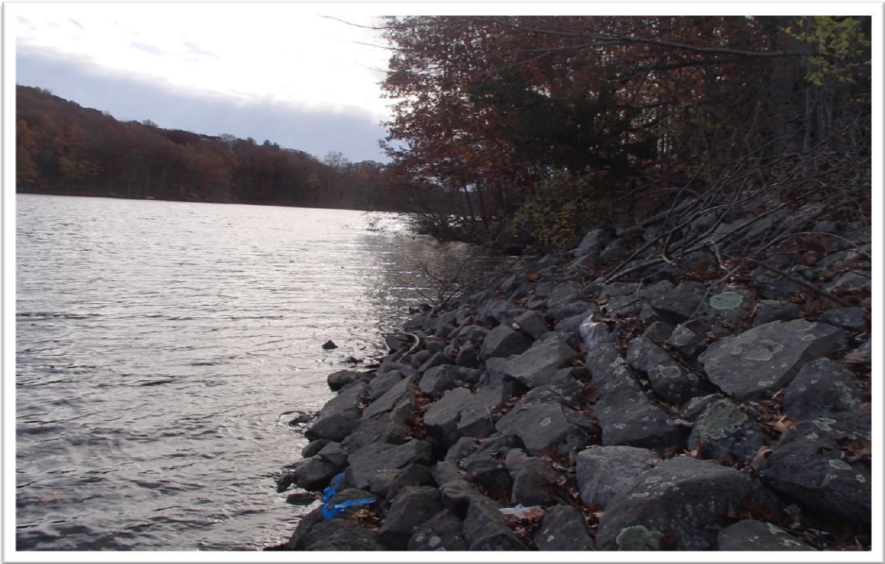
Photo A Baptist Church Road Bridge: View facing west showing non-wetland water edge of New Croton Reservoir along toe of roadway slope. Date Taken: November 7, 2018.
