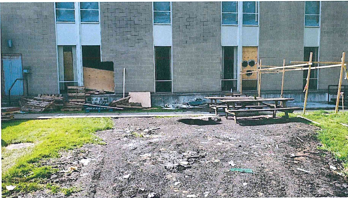
Photo 6 – Lower Level Demo
