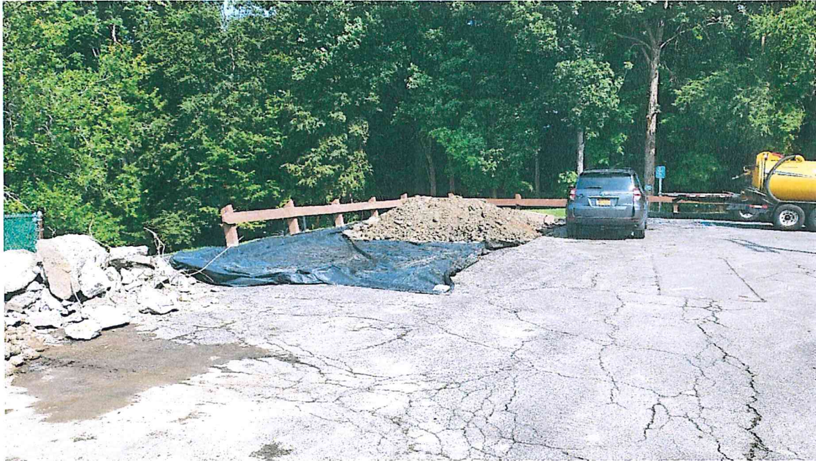
Photo 3 – Contaminated Soil Stockpile
