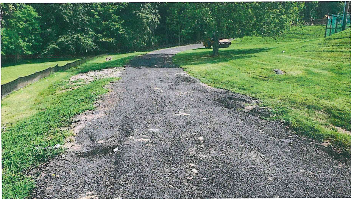
Photo 8 – Temporary Construction Access Road
