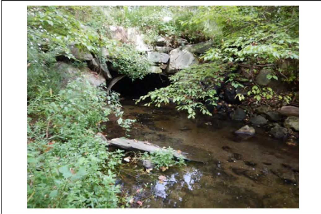
Culvert within Mohegan Outlet
