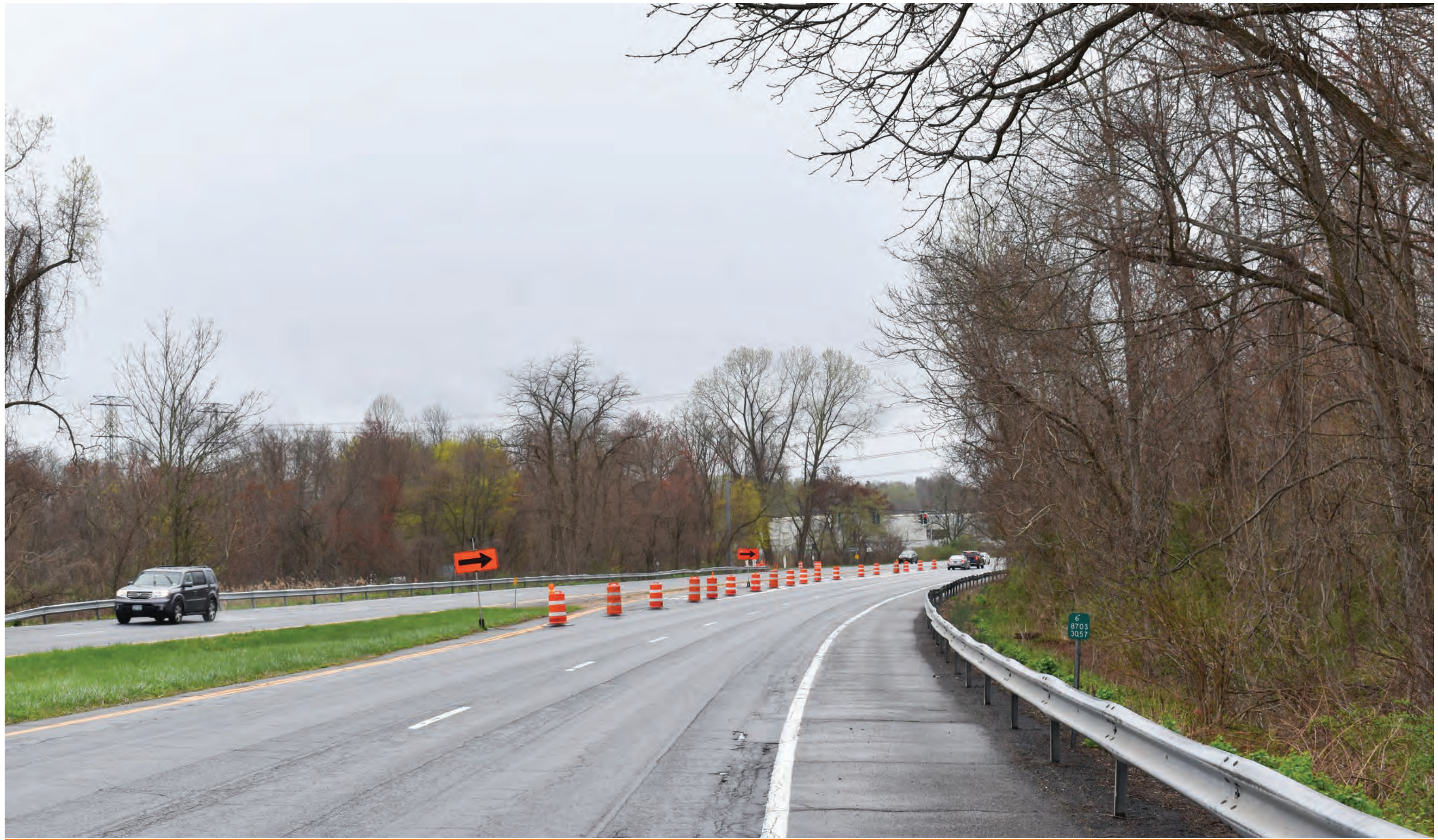
Photo 7 - Route 6 near Hill Blvd. EXISTING CONDITION
