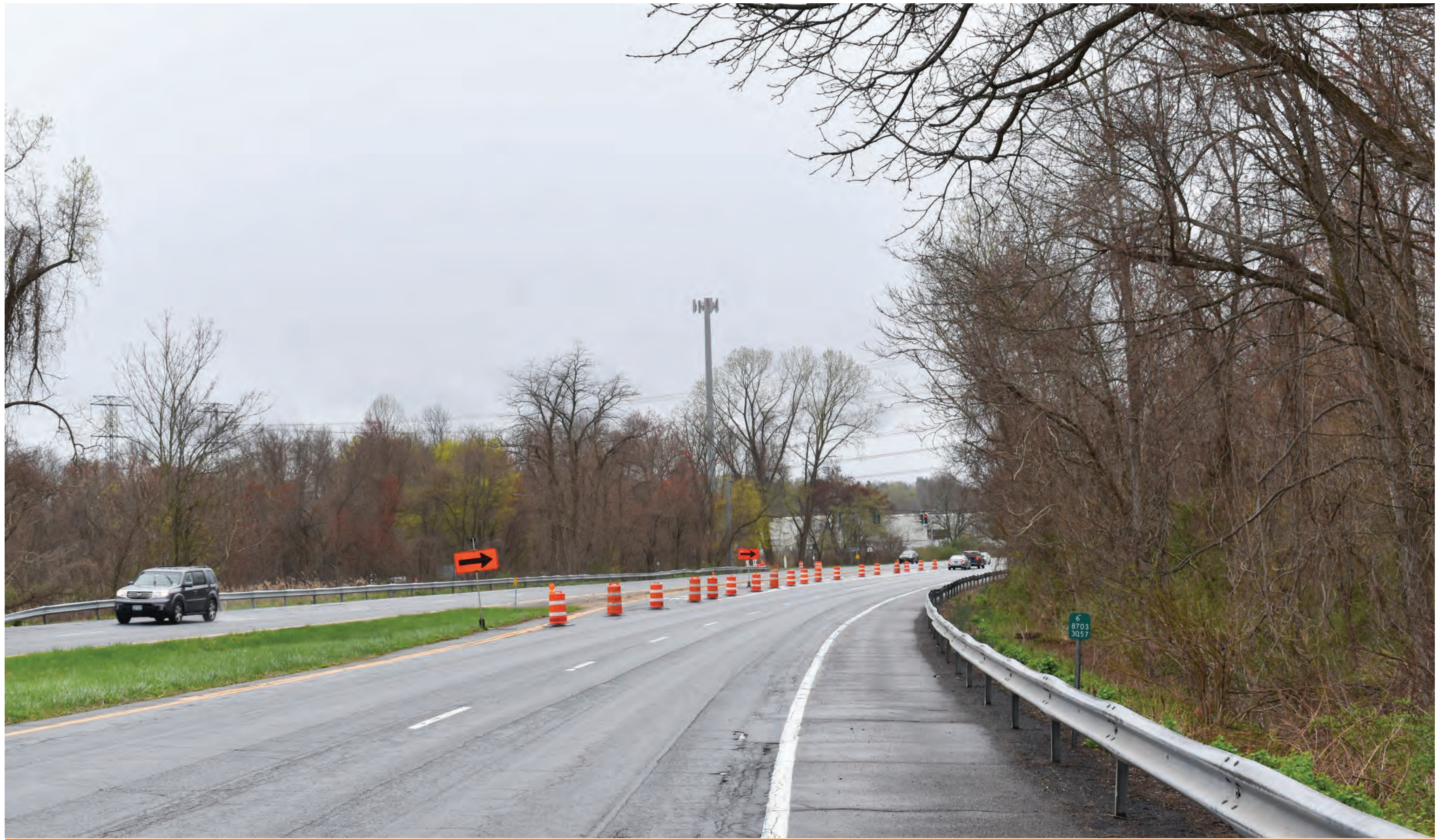
Photo 7 - Route 6 near Hill Blvd. SIMULATED CONDITION - 130FT MONOPOLE
