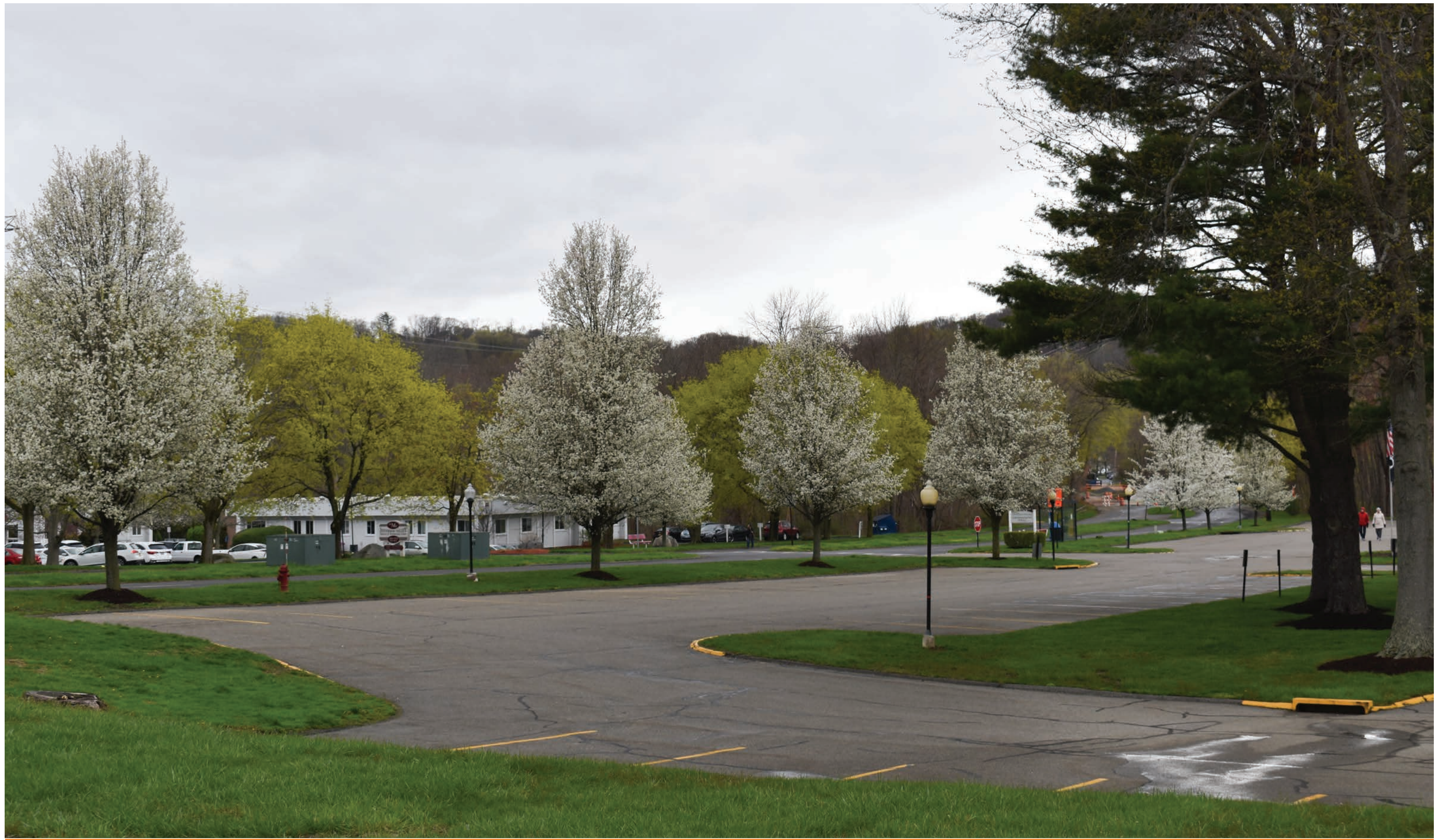
Photo 3 - Village Road near Hill Blvd EXISTING CONDITION
