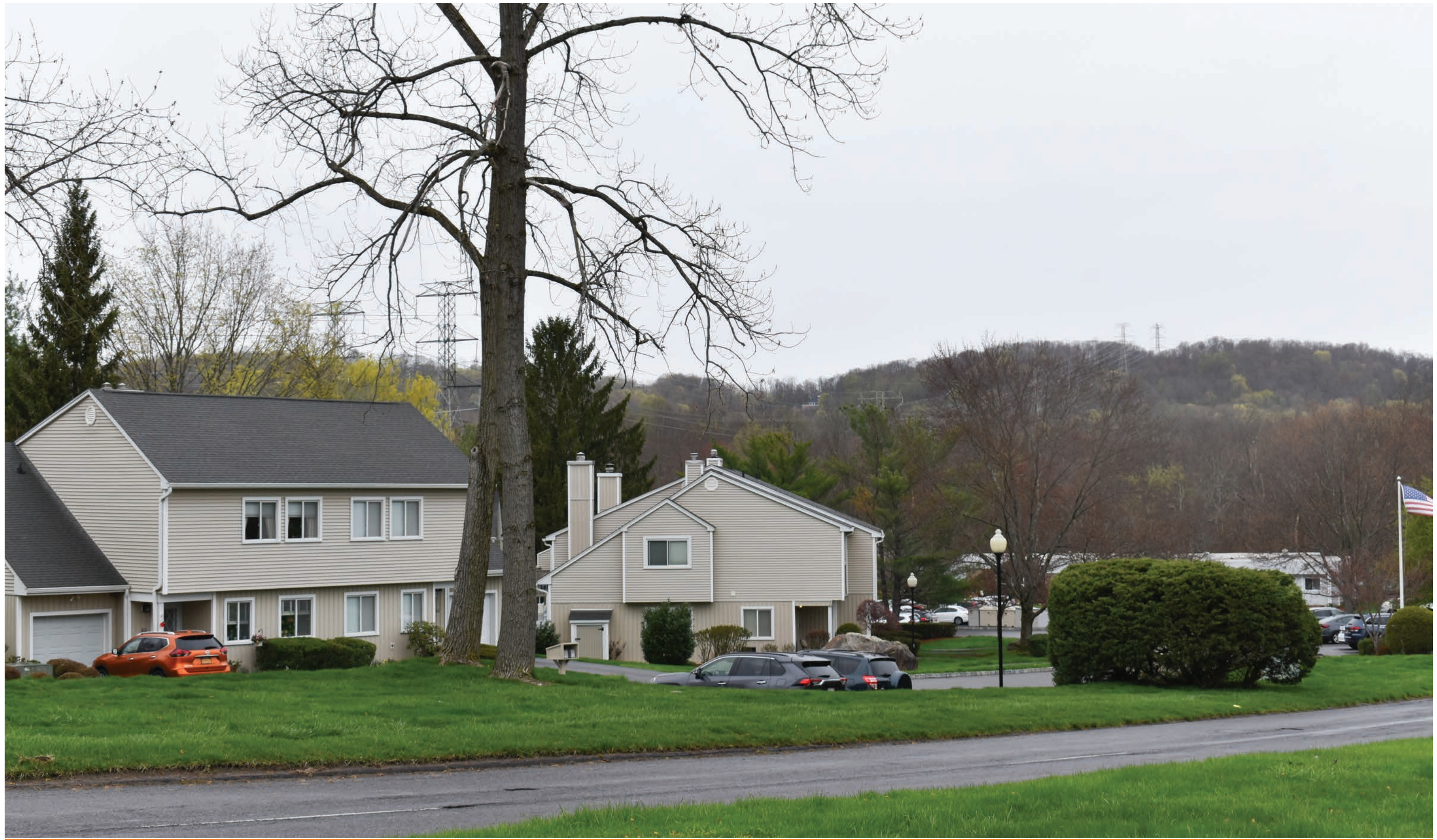
Photo 8 - Hill Blvd. near Lee Blvd. EXISTING CONDITION
