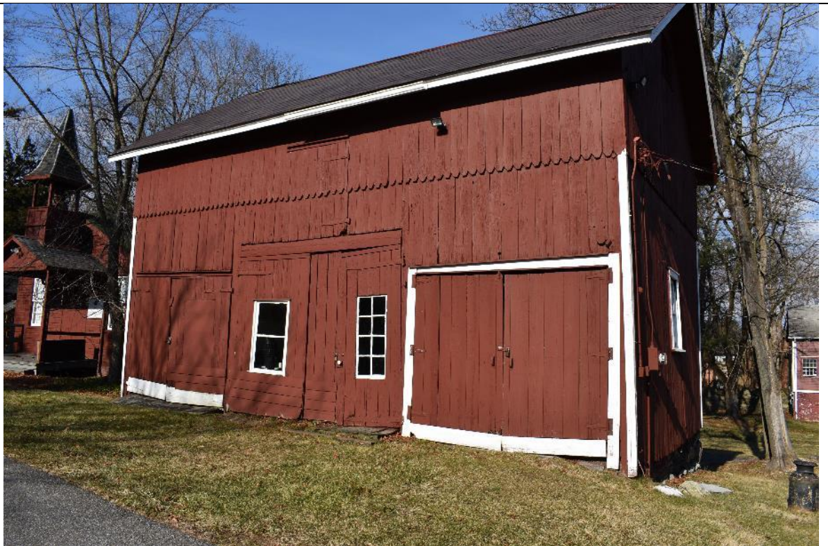
4. Building G was formerly a carpenter's workshop, and is used for storage.
