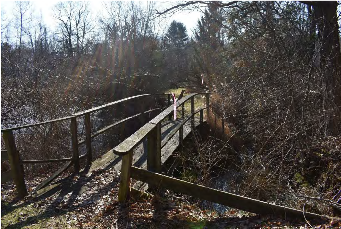
Photo 9: The pond drains to an underground outlet on the northern side of the pond. View to the southwest.
