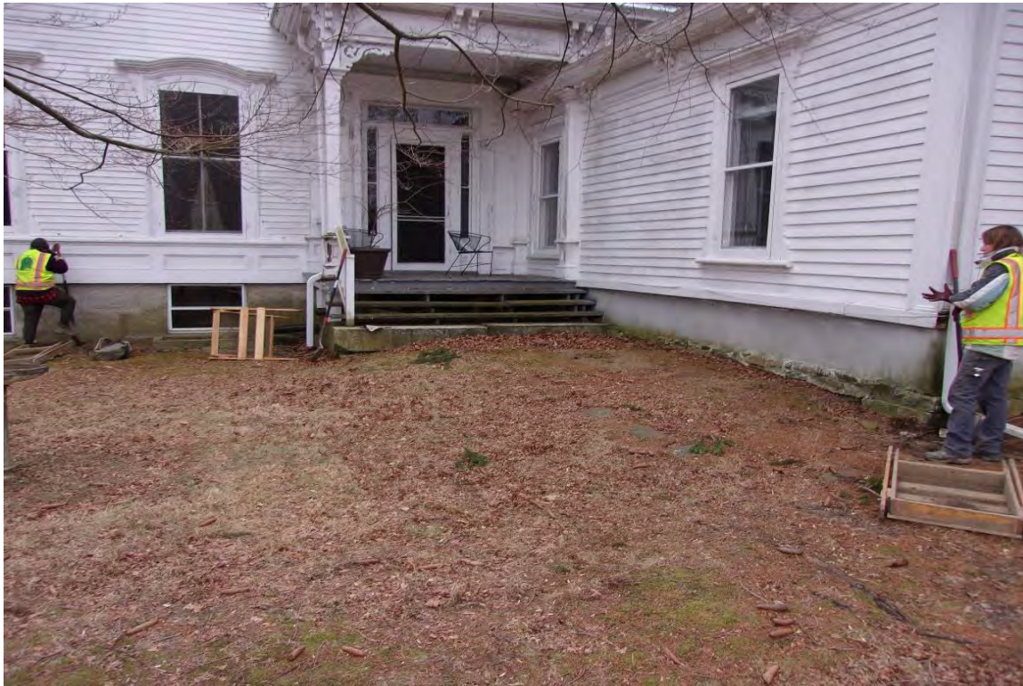
Photo 17: The perimeter of Building A was tested at 10' (3.04 m) intervals. View to the south.
