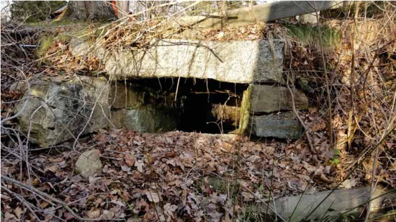
Existing Pond Outlet
