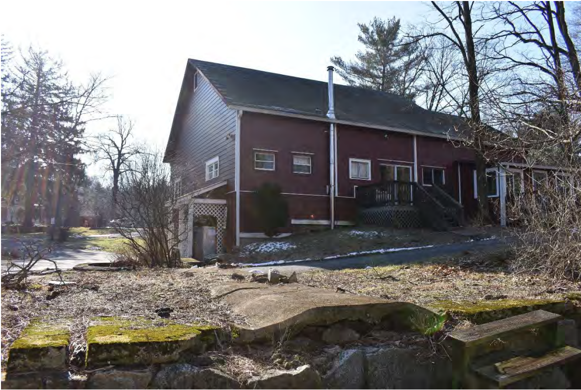
Photo 11: Portions of the foundation for Building D are visible on the landscape. View to the southwest toward Building E.
