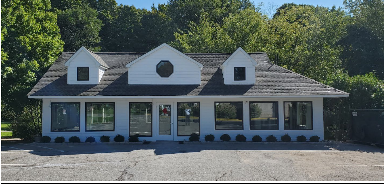
611 Granite Springs Rd, Yorktown Heights, NY - Carriage House
