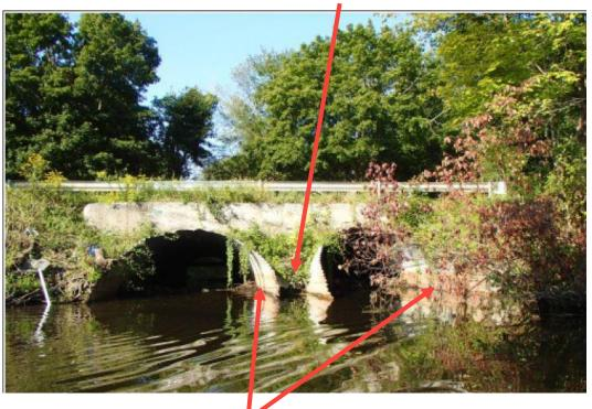
Significant corrosion and section loss of barrels - Yellow Flag Condition
