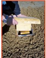
**Step Three:** Place the Soft Touch Base inside the receptacle (mount) with the yellow tapered plug inside.
