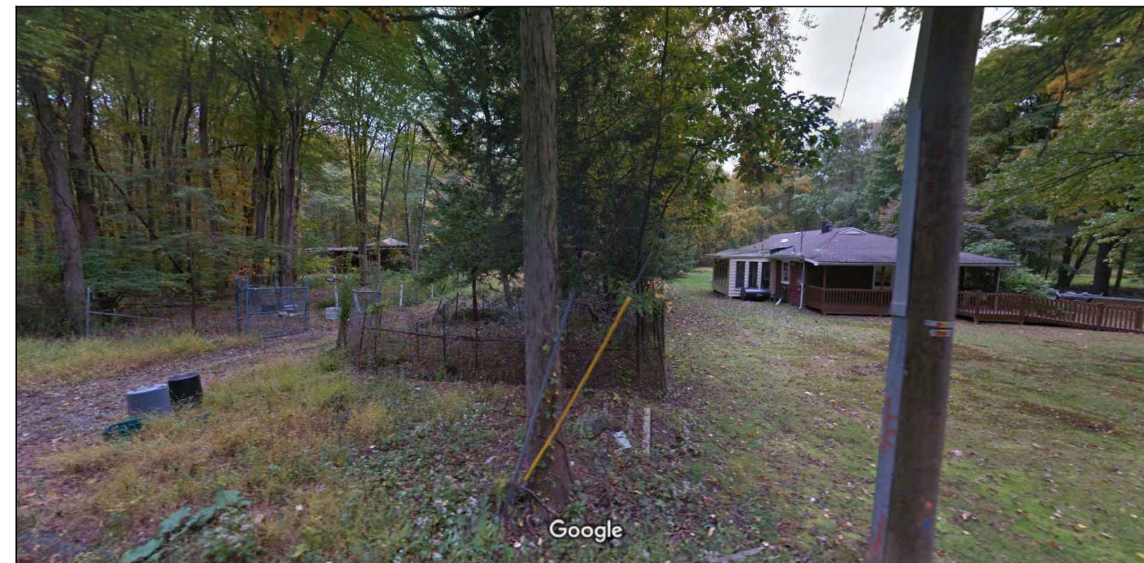
VIEW LOOKING UP NORTHERN PROPERTY LINE
