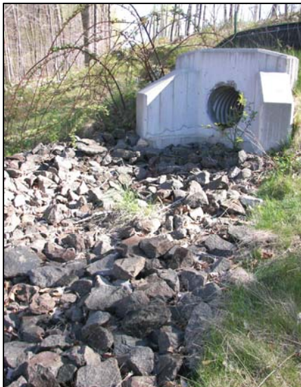
A drainage outfall.
