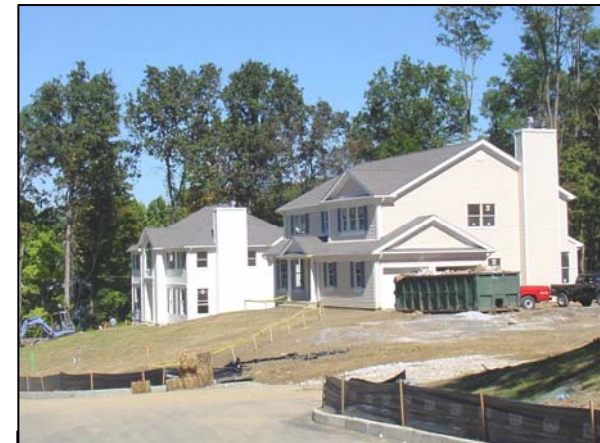
Erosion controls during construction of Kensington Woods Estates, Mohegan Lake.
