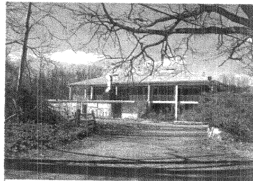
Exhibit III.B-4: Former motel on Project Site.
