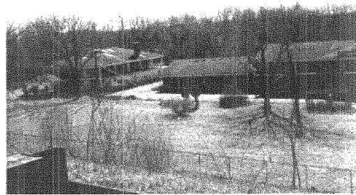
Exhibit III.B-12: View W from Taconic State Pkwy SB Ramp.
