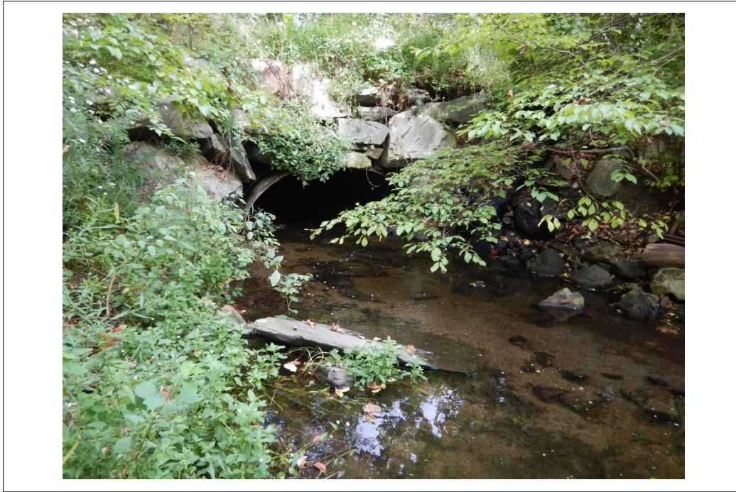
Culvert within Mohegan Outlet
