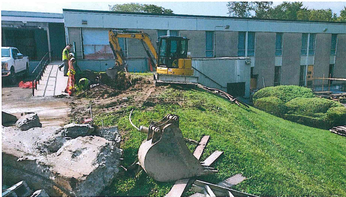
Photo 4 – Oil Tank Removal
