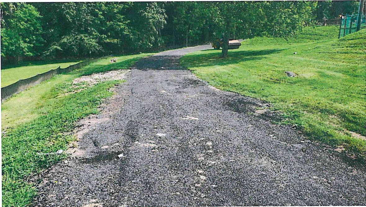
Photo 8 – Temporary Construction Access Road
