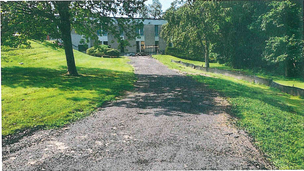
Photo 7 – Lower Level Demo and Temporary Construction Access Road
