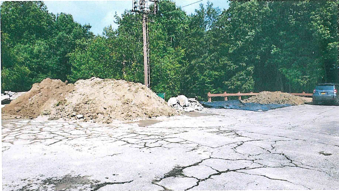
Photo 1 – Cut Material Stockpiles
