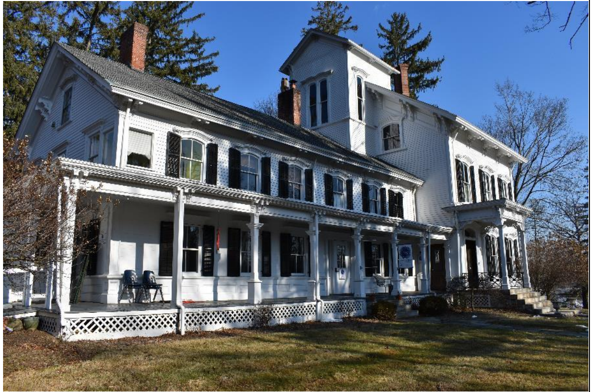
1. Underhill Estate/Sound view School (Building A). View to the northeast.
