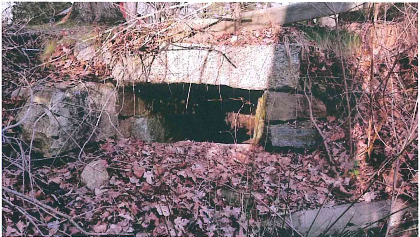
Existing Pond Outlet
