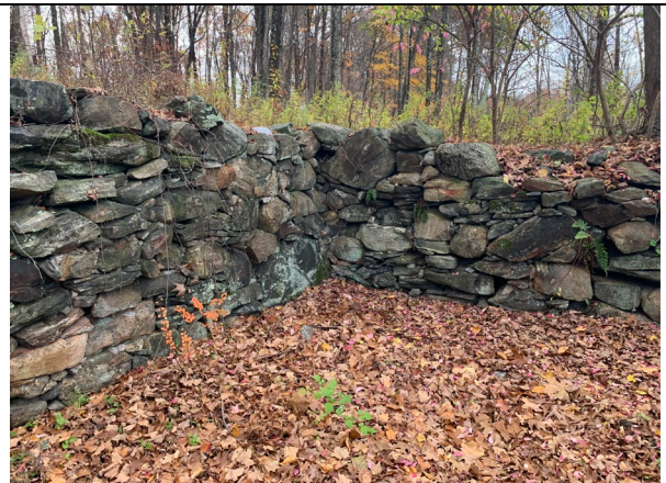
Photo 4: View of southeast area of the Site that previously contained three (3) aboveground storage tanks, three (3) drums, and approximately eight (8) containers likely containing petroleum-based liquids. The tanks have since been removed and there is no evidence of odor or staining.
