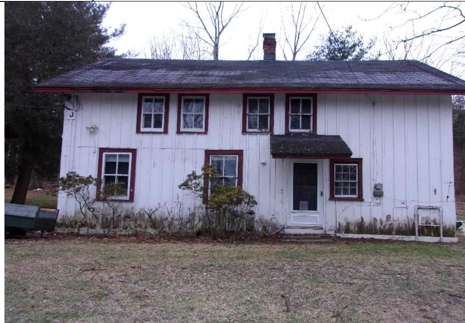
7. Building J, is a small residential cottage.
