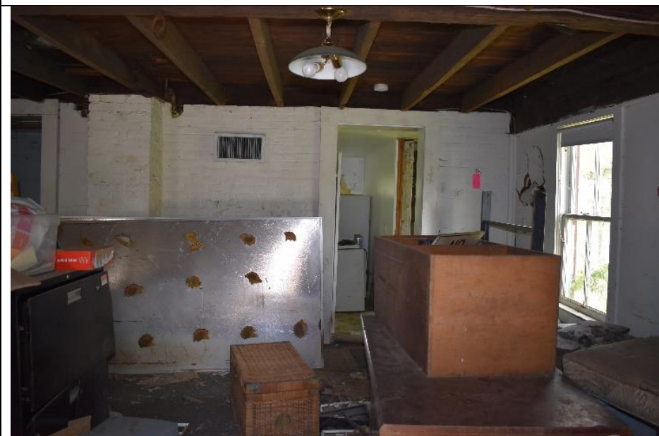
55. A brick wall divides the interior of Building J.
