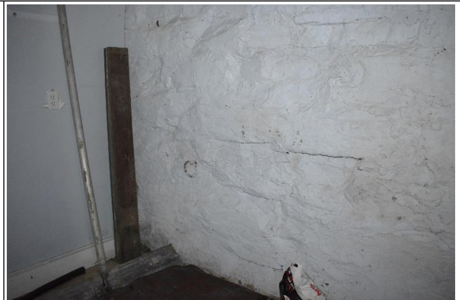
22. The northern foundation wall of Building E is the 19 th century stone barn wall, consisting of field stone that has been painted.
