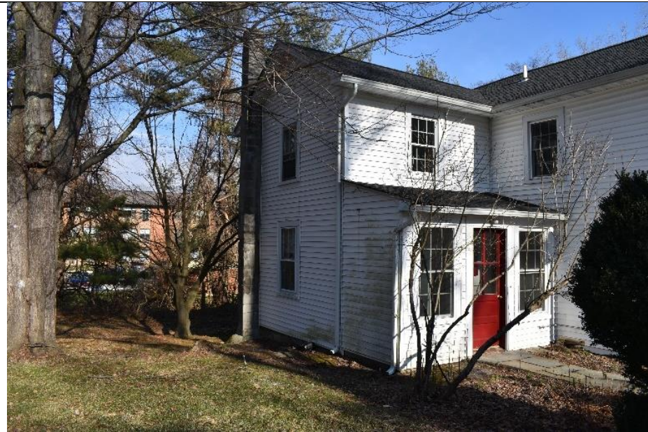
20. The western entrance of Building C features an enclosed doorway addition.
