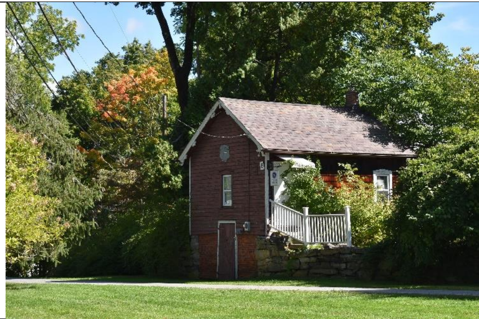
13. View to the northeast to Building B.
