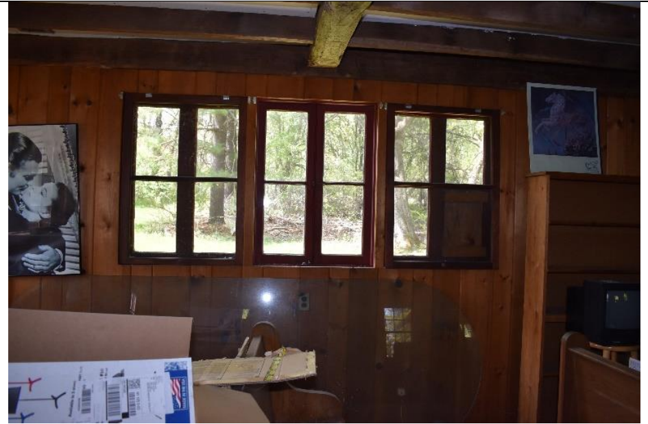
50. The windows of Building I are a mix of double hung and casement styles.
