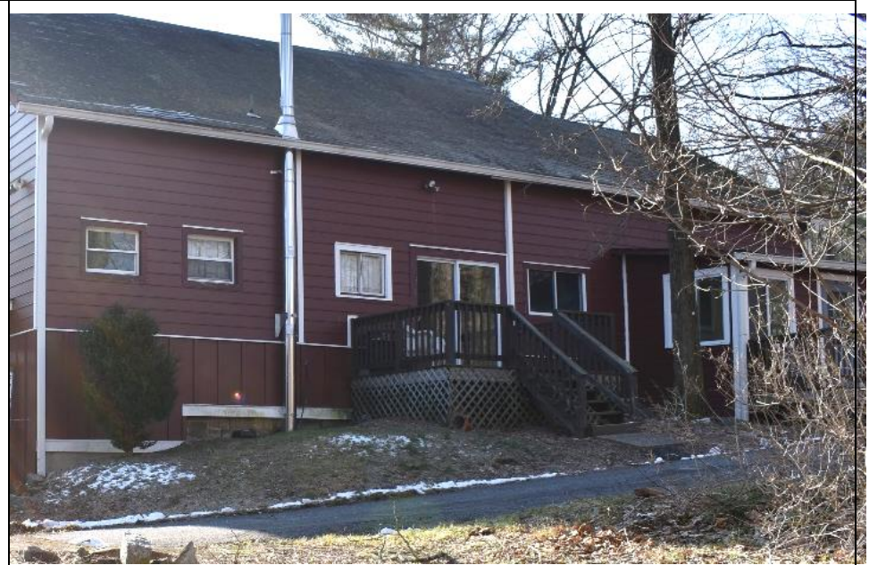
30. The rear entrance of Building E has been altered and includes modern sliding glass doors and windows.
