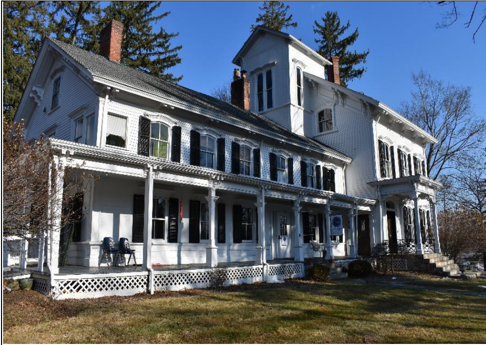
1. Underhill Estate/Soundview School (Building A). View to the northeast.
