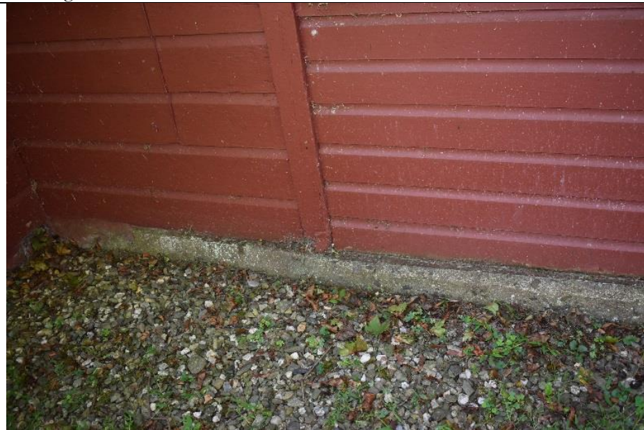
47. Building H is located on a poured concrete slab.
