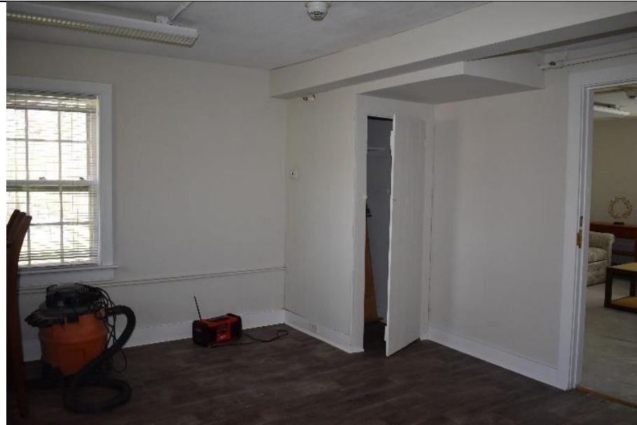
17. The interior of Building C dates to the mid 20 th century.
