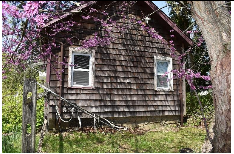
16. The windows are modern vinyl replacements, and the siding style differs on the exterior.
