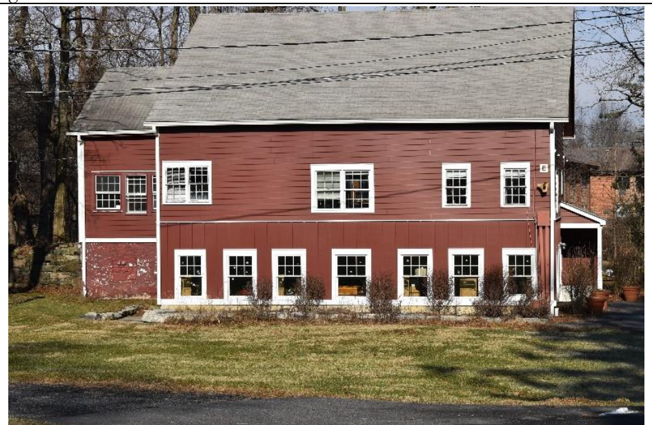
32. Building E- The windows on the first level of the southern elevation are all modern vinyl replacements, and the second are irregular in placement.
