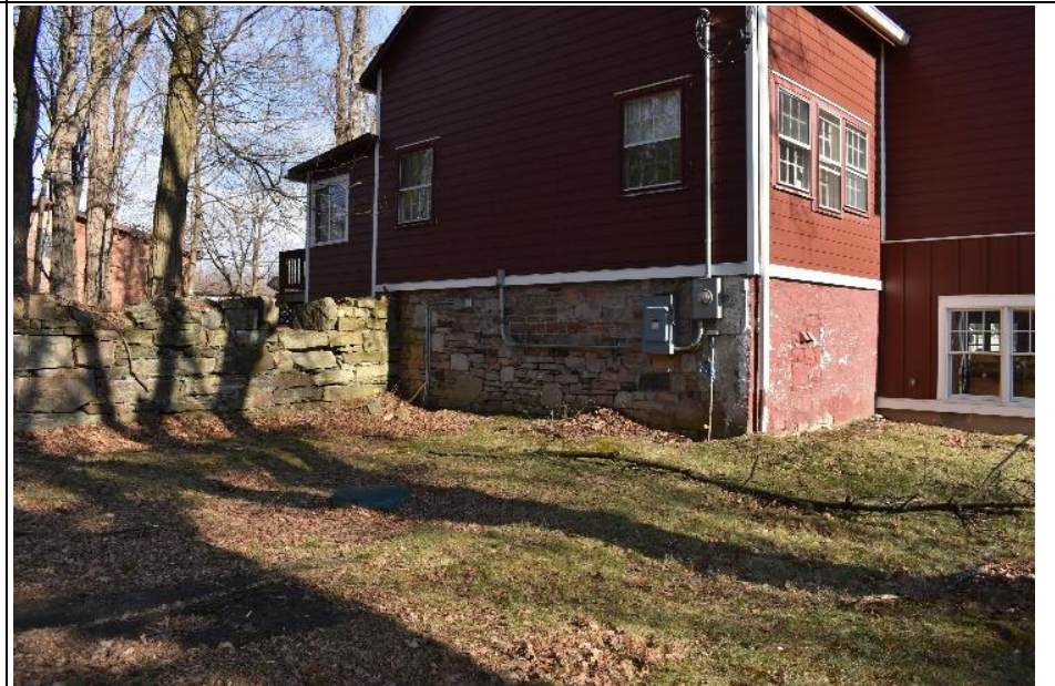
28. Portions of the western foundation wall of Building E have been reconstructed using stone, possibly from the original barn.
