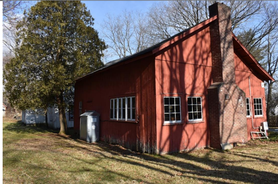
9. View to the northeast of Building I.
