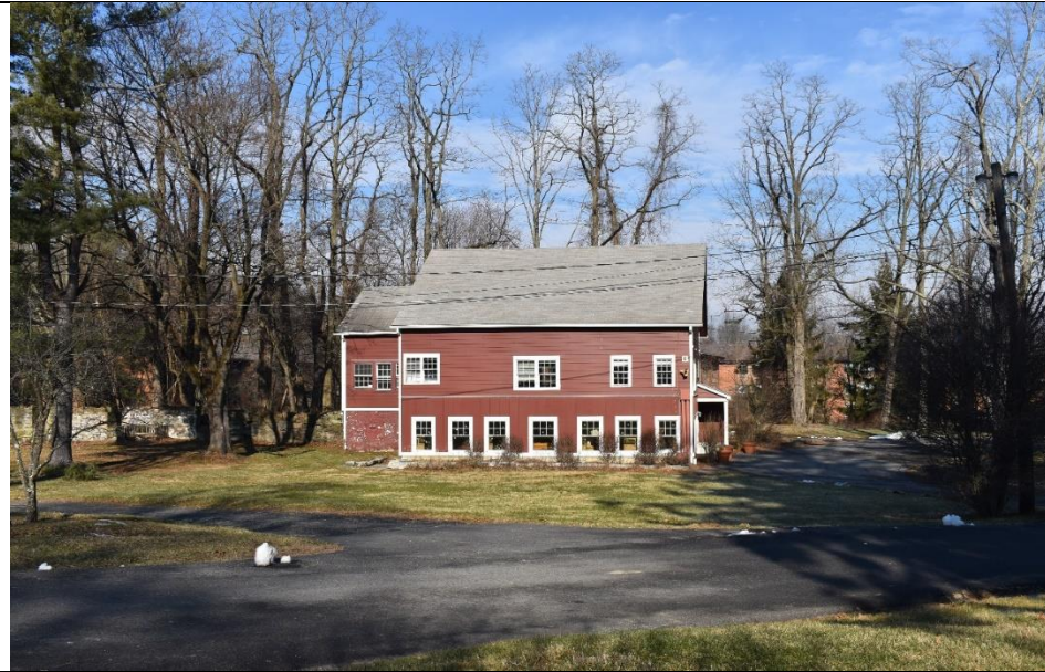
5. Building E is the Science building. This structure, formerly the carriage house, was substantially rehabilitated in 2012.
