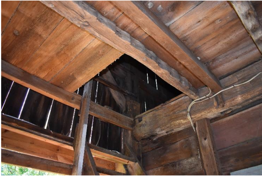
41. The interior of Building G is a mix of timber and 20 th century lumber. Cut outs and openings in the timber are indicative of reuse.
