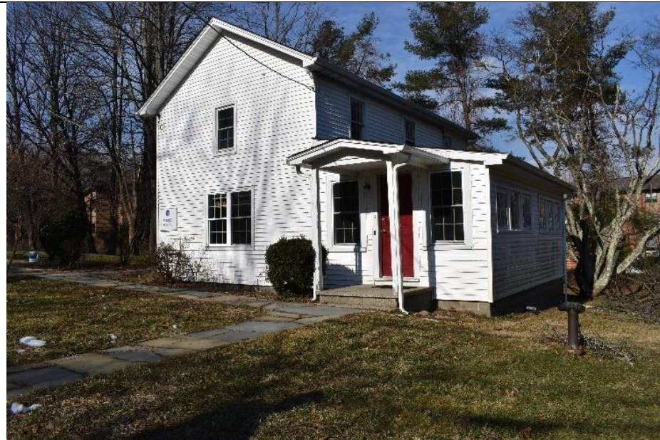
19. The exterior of Building C includes modern vinyl siding.
