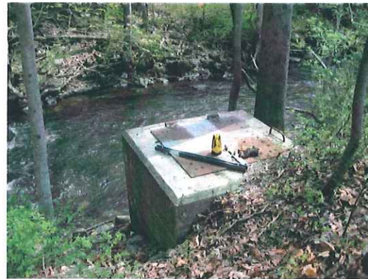
Photograph 1: Hunters Brook Steel Pipe Siphon east blow-off chamber at Hunter Brook.
