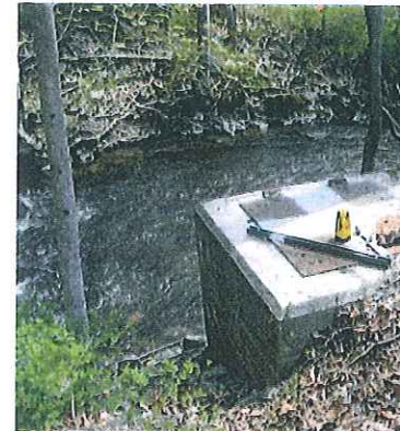
Photograph 1: Hunters Brook Steel Pipe Siphon east blow-off chamber.
