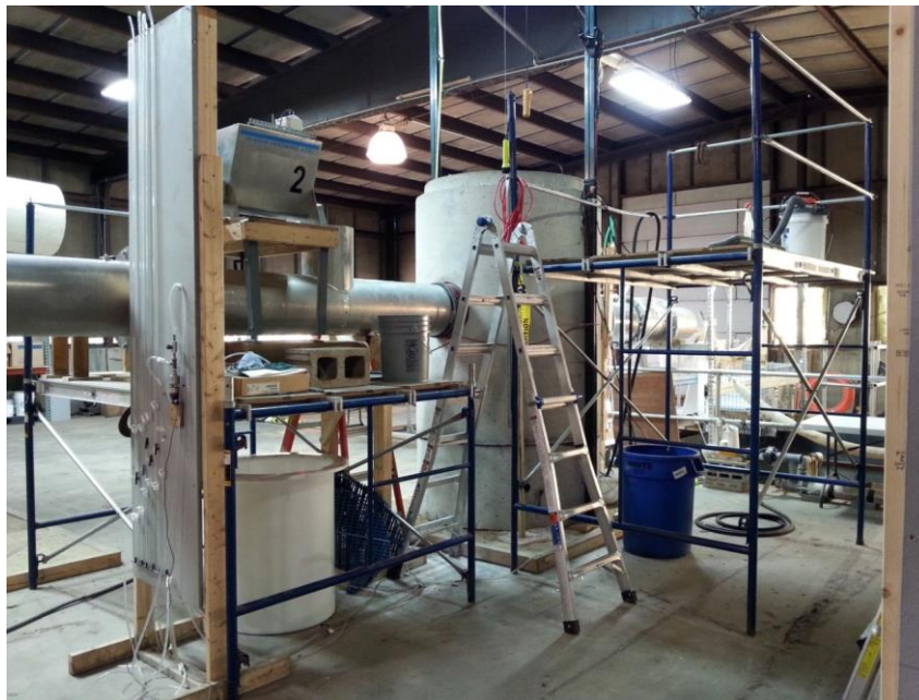
Figure 3 Photograph of HS 4 Test Unit Installed in Alden Test Loop
