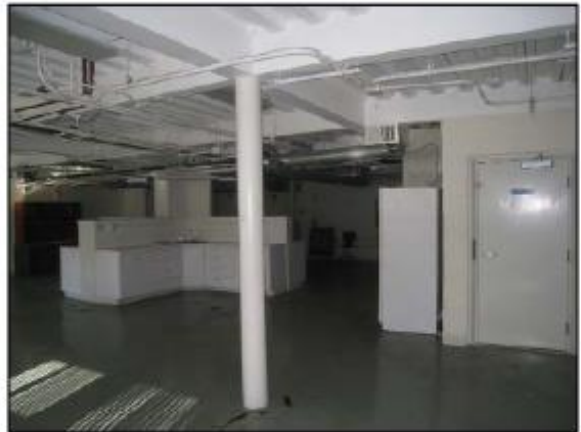
Open Basement Area
