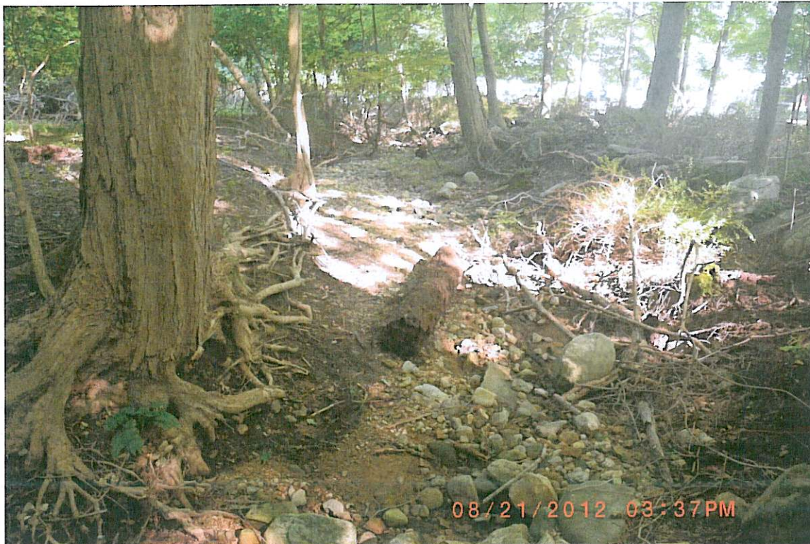
Photo 2 - Example of severely eroded and sediment laden Forested Intermittent Watercourse (FIW).
