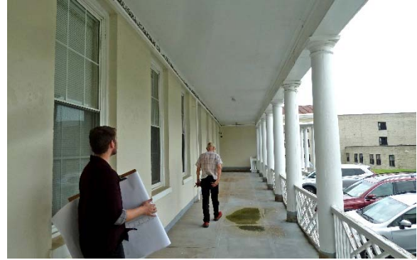
South porch: replacement balusters, coated floor and Tuscan column bottoms; bird deterrent visible above windows
