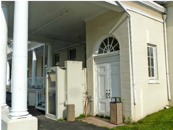
Primary access to first floor provided by stairs and lift to south porch, and Chapel entry, on grade, along the South Elevation
