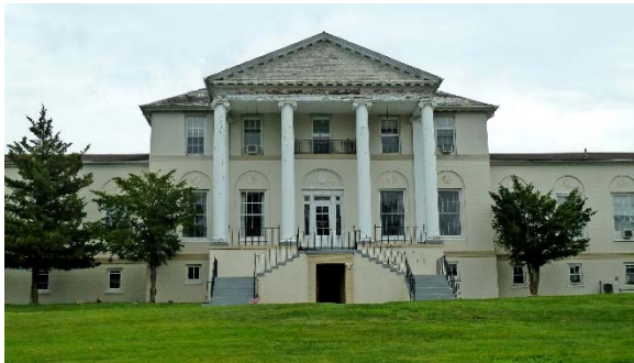
West Elevation, 1924 addition, grand entry with pedimented portico, Ionic columns, grand staircase, & Basement entry
