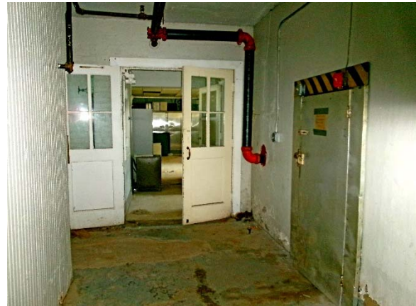
Central hall looking towards kitchen in East Pavilion, with door to mechanical room beneath the Chapel on the right
