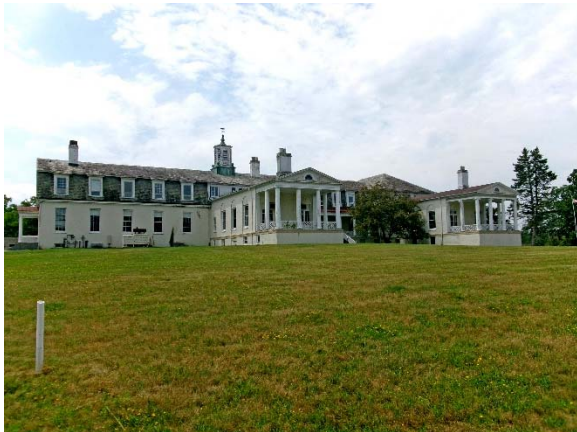
North Elevation including 1889 Chapel (left) and pair of 1924 pavilion additions with open porches
