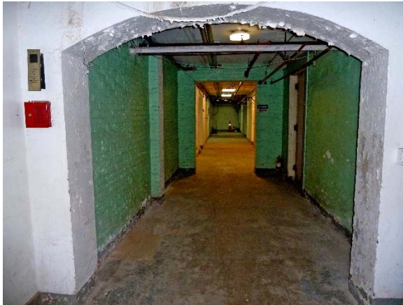
Central hallway inside exterior entry, looking eastward to Chapel basement/mechanical room
