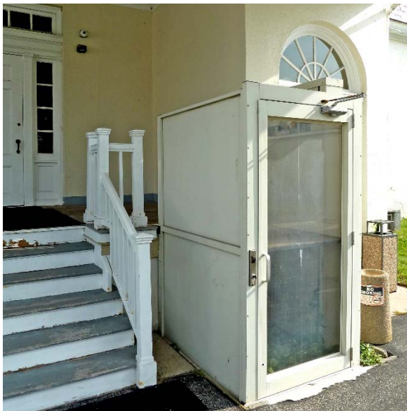
Stairs and lift (possibly inoperable) beneath entry portico, providing access to porch/first floor level
