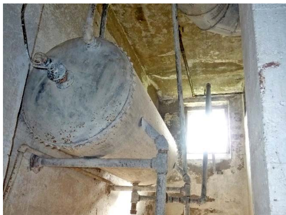
East Pavilion basement: likely remnants of 1924 systems
