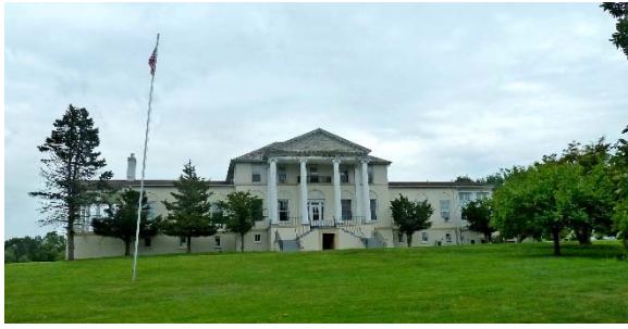
West Elevation, 1924 addition, as viewed from the lawn and Catherine Street
