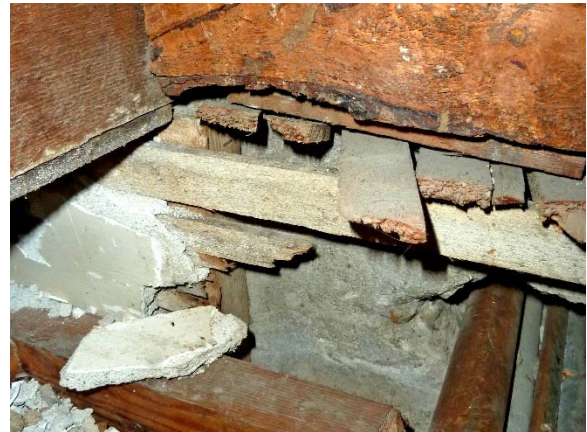
Kitchenette: floor probe exposes plaster walls above a dropped ceiling, and concrete wall penetration
