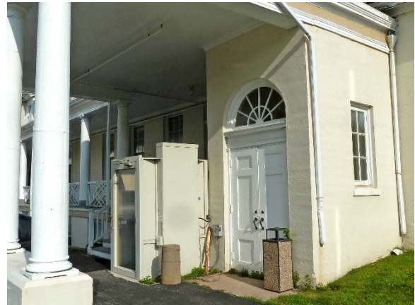
Entry portico (1924 Addition): lift to porch/first floor level adjacent to vestibule leading to Chapel (all beneath roof)
