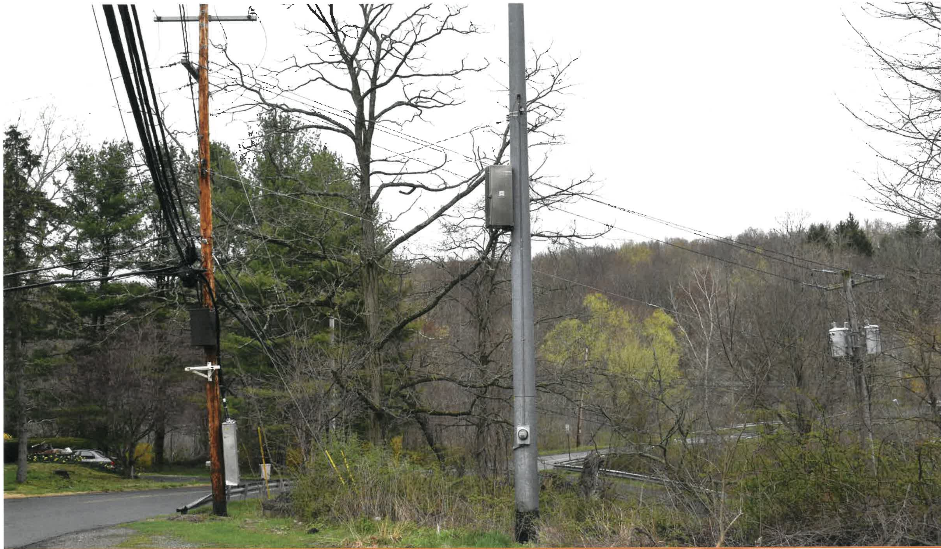
Photo 1 - Granite Springs Road EXISTING CONDITION
